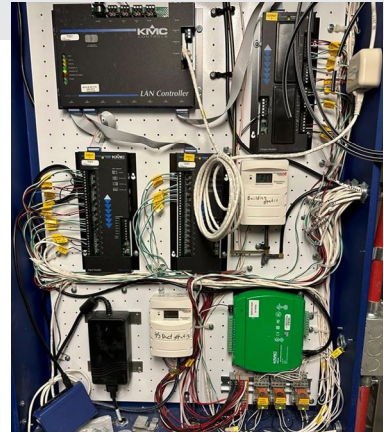
Data integration with the AFMS (green) was achieved through BACnet/IP over Ethernet.
