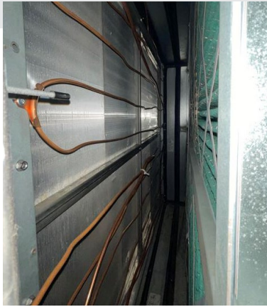
Outside, return, and mixed air (pictured) temperature sensors were installed.
