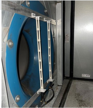
Airflow measurement probes were installed on the supply (pictured) and return fans.
